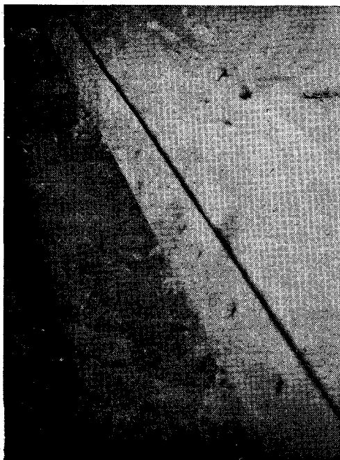
Fig. 1—Plugging of superheater tubes by vanadium rich deposits.
