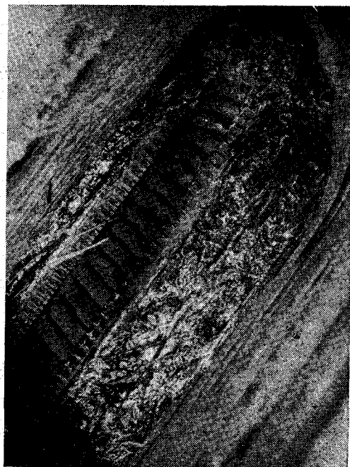
Fig. 2—Return bend of superheater covered with deposits.
