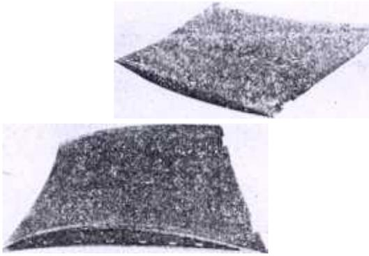
Figure 7. Hollow vane constructions via DB/SPF.
