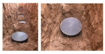
Figure 4. Placement of the pressure transducer.
