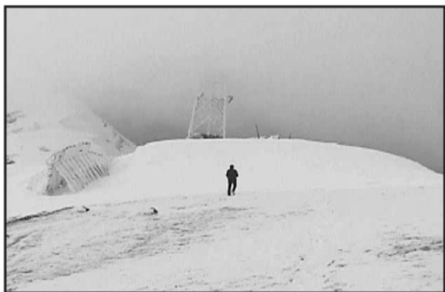
Figure 5. Snow deposition profile on back side of snow fence.
