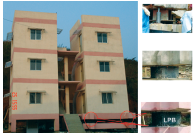
Figure 5. Prototype base isolated and conventional structure at gauhati and installation of base isolators (P.N. Dubey, 2007).
