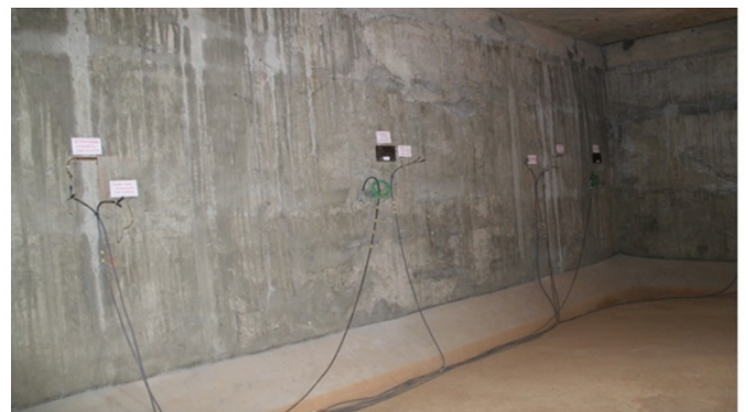
Figure 9. Deployment of sensors inside acceptor compartment.
