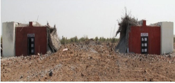
Figure 11. Structure after the blast.
