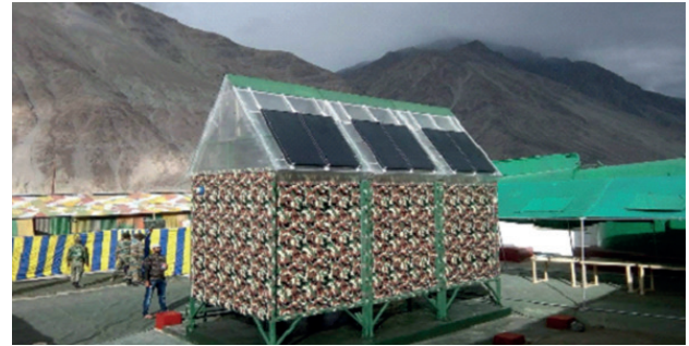
Figure 12. Completed and installed SILO at Khalsar, Ladakh.
